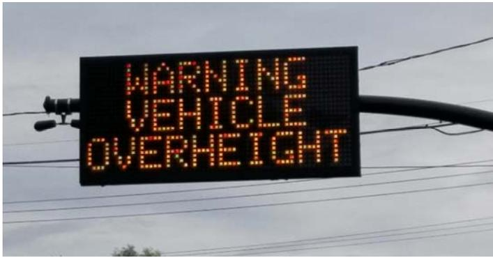
The laser-activated advance warning system activates when vehicles exceed the posted height. The state of Ohio paid for the system and City staff did some of the installation work. It was completed under budget in late 2018 for \$165,000.
