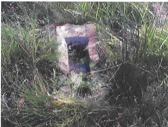
Figure 2 - 6 inch Pipe outlets and Concrete Collar
